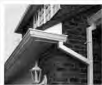
Fascias, Soffits and Guttering
