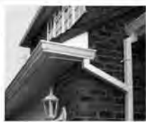
Fascias, Soffits and Guttering
