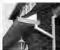
Fascias, Soffits and Guttering
