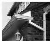
Fascias, Soffits and Guttering
