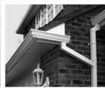
Fascias, Soffits and Guttering
