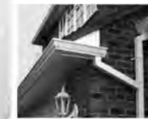
Fascias, Soffits and Guttering
