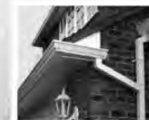
Fascias, Soffits and Guttering
