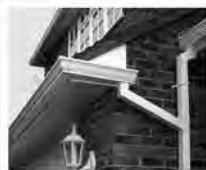
Fascias, Soffits and Guttering
