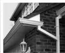
Fascias, Soffits and Guttering
